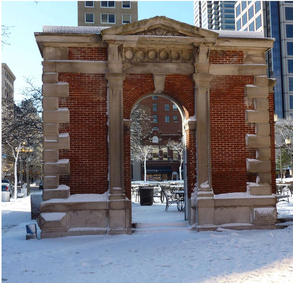
Figure 0.A: The only remnants of Tomlinson Hall are this arch, outside of the east wing of the Market House. This arch was discovered and saved during the 1979 renovations. A bronze plaque on opposite side gives a brief history of Tomlinson Hall. Photo by author.
