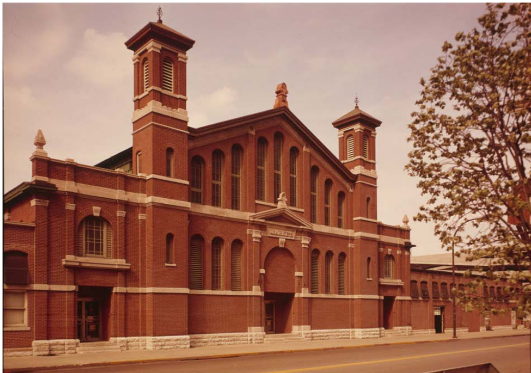
Figure 2.B: After the Tomlinson Hall fire in 1958, the city added sheds to the remaining Market House. This accommodated vendors displaced from the fire. Library of Congress, 1970, Historic American Buildings Survey, Indianapolis City Market , Survey HABS IND-59.
